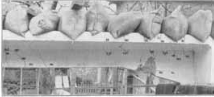
Figure 3. Experimental research of a continuous beam with crack pattern.
